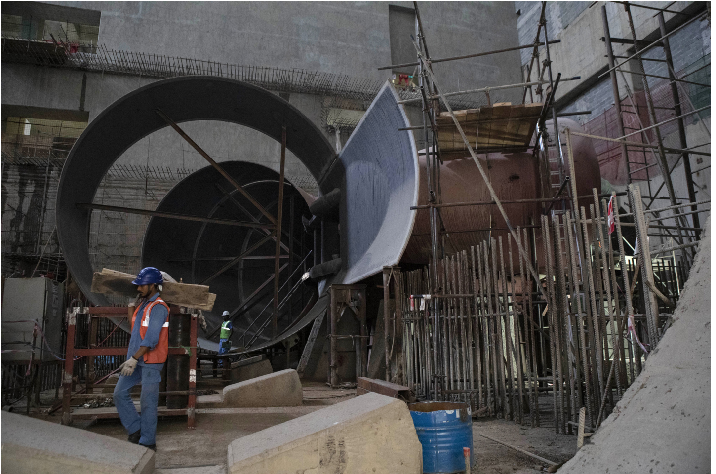
Top: The spillway that allows water to flow out of the reservoir when it overfills. Bottom: Part of piping that will direct water into the turbines. Photographer: Zacharias Abubeker/Bloomberg
